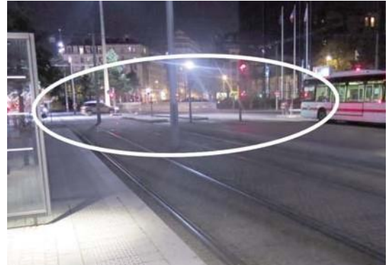
In the absence of special lighting of the trackbed, visibility on pedestrian crossings is sometimes insufficient
