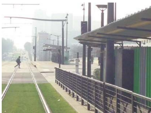
Site protection masking other users and signage
