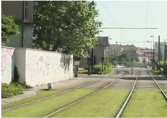
The wall close to the trackbed and the road makes it impossible to see whether a vehicle is stopped behind the R24 signal and mobile barrier
