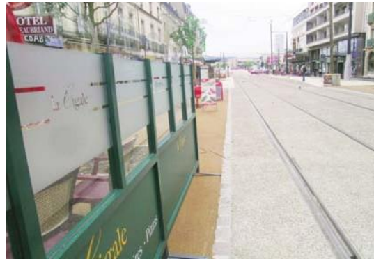
Bar or restaurant terrace windbreak that may hide a pedestrian wanting to cross the trackbed
