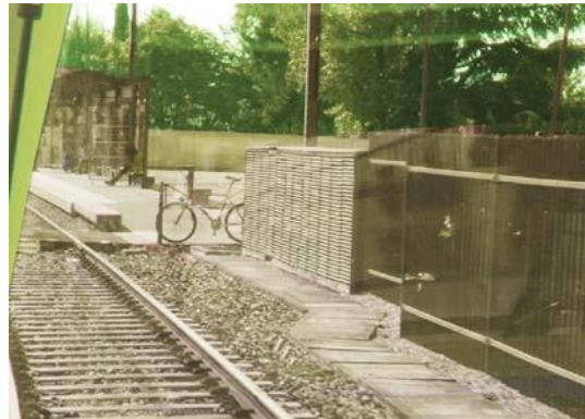
Pedestrian crossing obscured by the electrical cabinet
