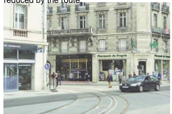
Building angle preventing the tram driver from seeing pedestrians waiting to cross
