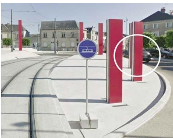
The artwork on the roundabout compromises visibility between trams and other vehicles
