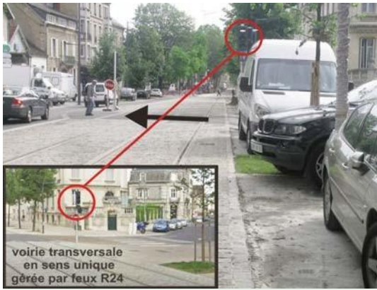
Difficult for the tram driver to see what traffic is on the adjacent road
