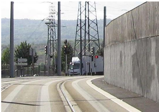
Retaining wall masking signalling in the bend
