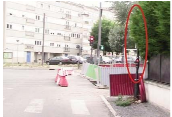
Mask detected during work to build the trackbed: resident hedge obscuring the traffic light
