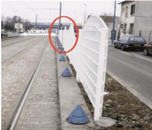
Poor visibility of the break in the barrier and therefore of any pedestrians likely to cross the trackbed
