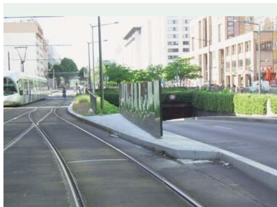
Anti-glare device between tram trackbed and road
