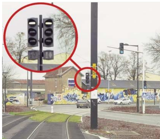
If it were not duplicated, the R17 signal would be obscured by the overhead power line post
