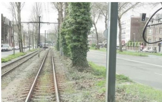
Alignment of plants affecting the tram driver's visibility of any unauthorised crossing of the trackbed by pedestrians
