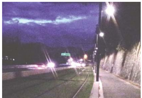
The position of the trackbed parallel to the road can cause reciprocal glare problems due to the lack of residual or urban lighting.
