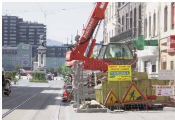
A building near the minimum clearance outline requires consultation
