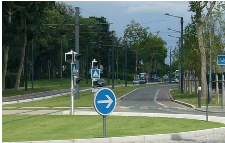
Photo 18: Repeating the R24 barrier signals allows optimising their perception by all users (source: Cerema)
