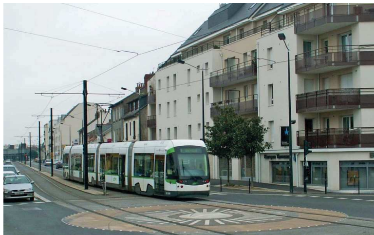
Photo 11: marking of the central traffic island of a mini-roundabout (source: Semitan)
