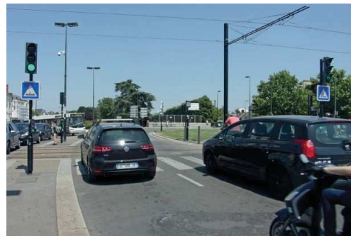
Photo 20: repetition of signals at a crossing of a roundabout branch (source: Cerema)
