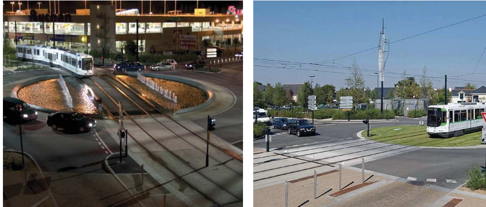
Photos 9 and 10: marking of the platform to enhance the perception as compared to the circular road (source: Semitan)
