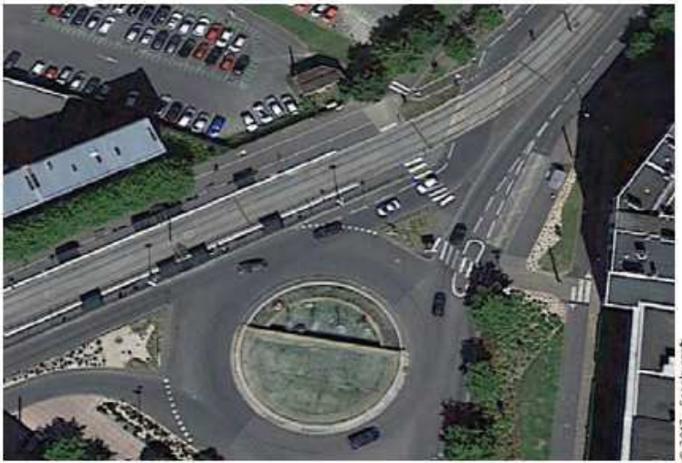
Photo 12: marking of the platform crossing a branch of the roundabout
