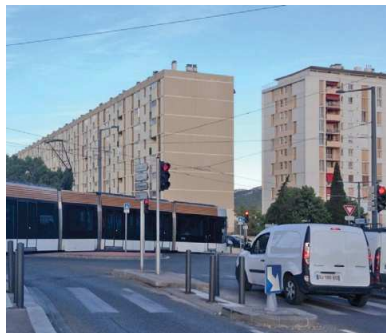
Photo 19: the presence of a traffic island enables repeating the R11j signal at the entry of the roundabout (source STRMITG)
