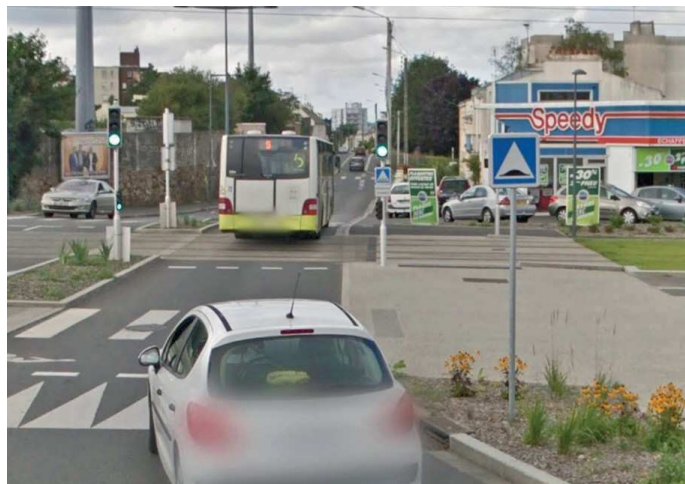
Photo 17: R11v barrier signals at a crossing of a roundabout branch
