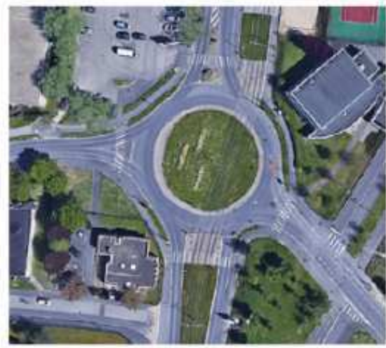
Photo 3: the lateral positioning on the north branch is acceptable, given the wide angle with the previous branch.
