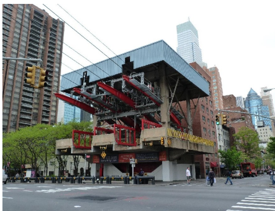
Aerial tramway station of Roosevelt Island in New-York (photo CETE of Lyon)
