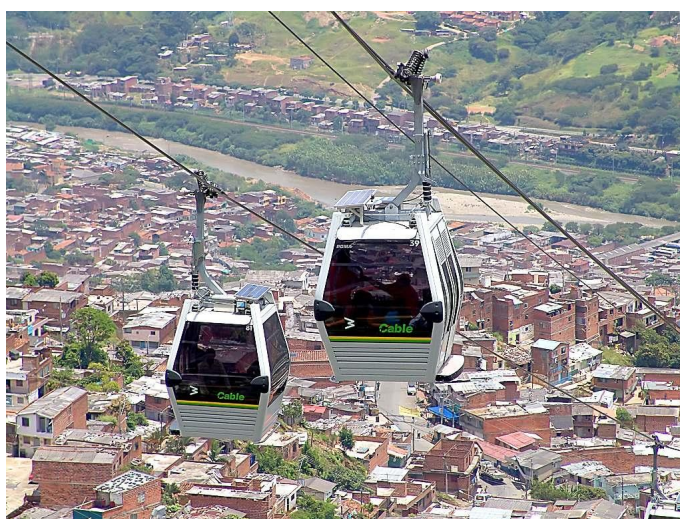
The CableTrain in Medellín takes is helping to open up and develop some of the city's neighborhoods (photo Pomagalski)
