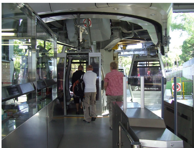
Barcelona : speeds are reduced to make boarding easier at station (photo Anne Le Ruyet – CETE of Lyon)
