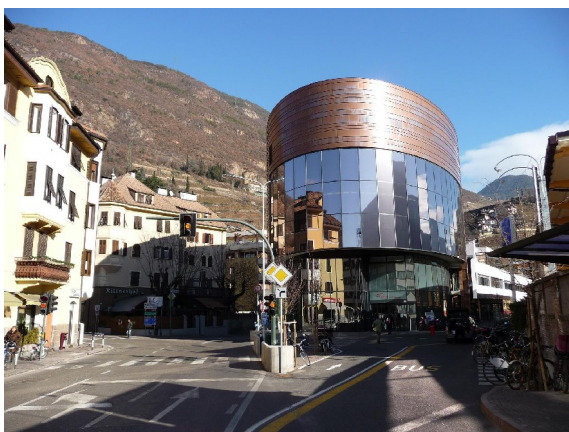
Lower station on the bicable gondola in Bolzano (photo Leitner)
