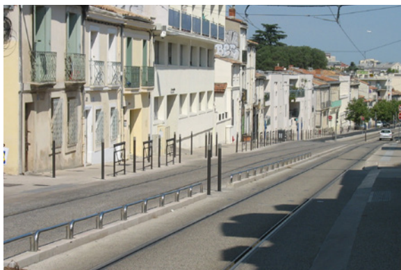
Illustration 3: Separators upstream of a staggered platform station in Montpellier
